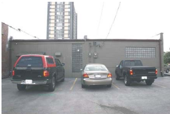
View of Subject Property – Rear Elevation
